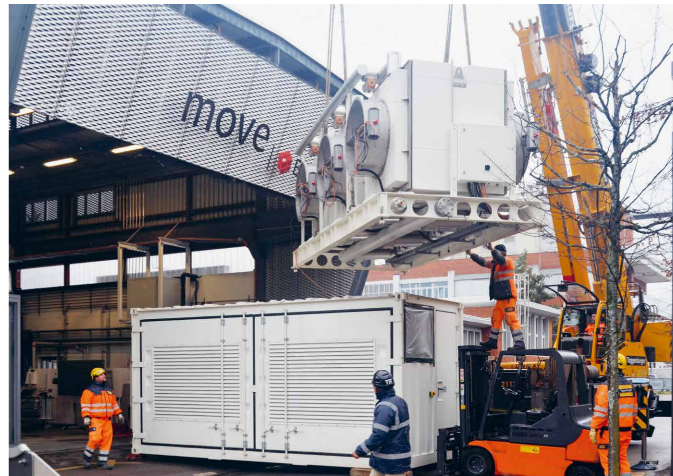
Special delivery for move: at the end of November 2021, a Climeworks direct air capturing system was delivered to the Empa mobility demonstrator. This system collects CO 2 from the atmosphere that is used for the production of synthetic methane in a further step.
