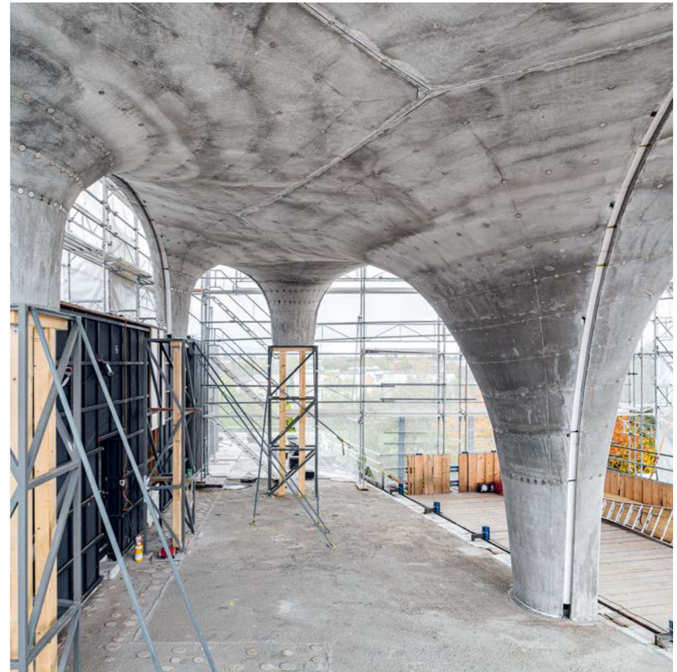
Concrete was sprayed on a textile shell for the roof of the “HiLo” unit. Image: Roman Keller
